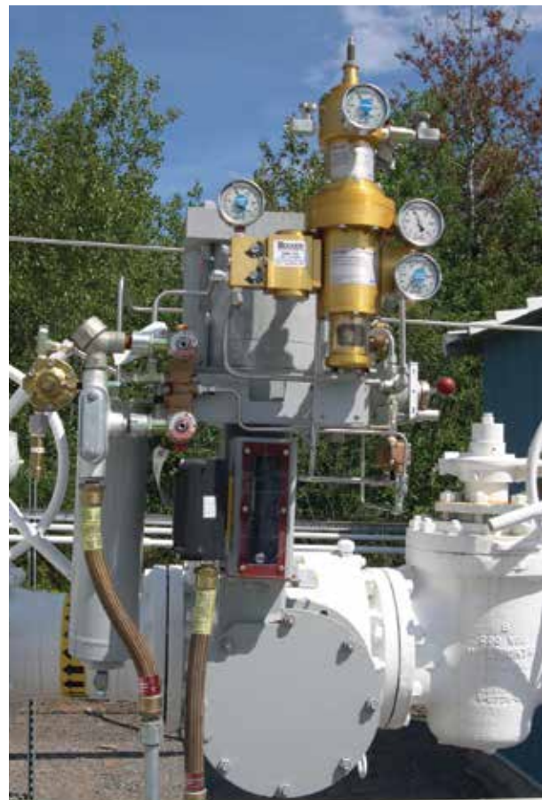
Figure 9- Model VRP-B-CH Pilot with Electrical Override
