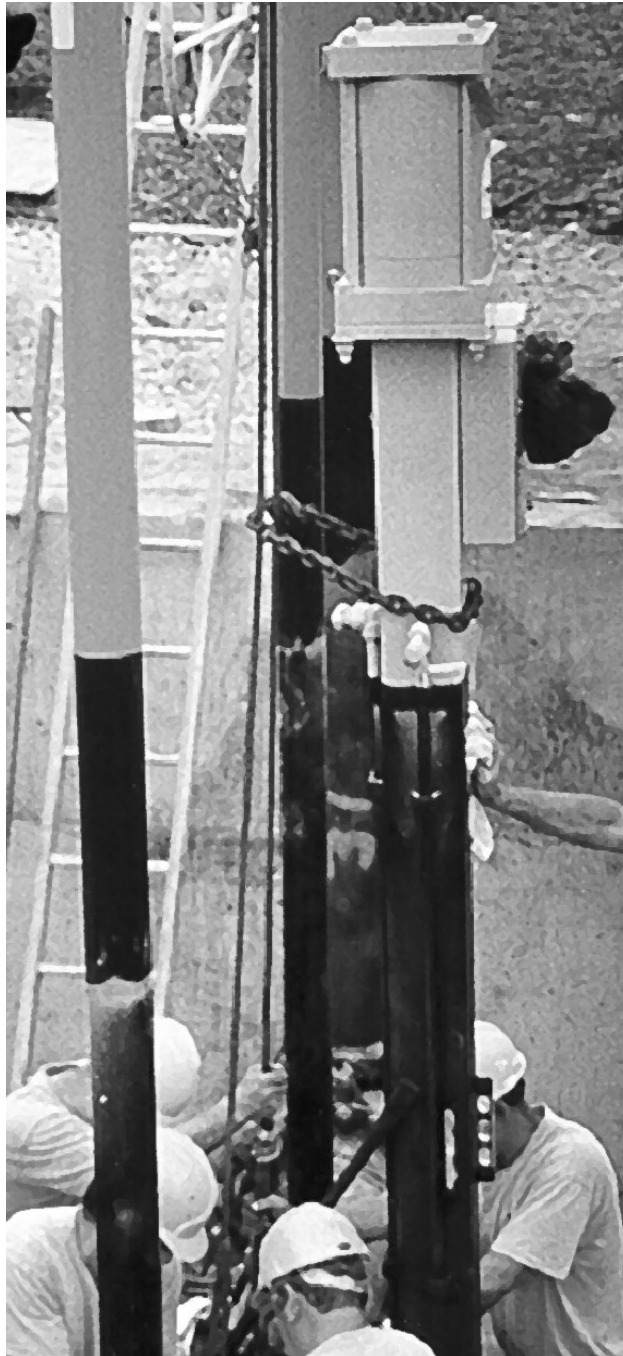
Figure 1.0 Installation of Becker Below Ground Ball Valve Regulator.
