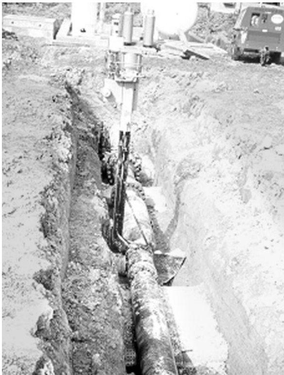
Figure 2.0 Below Ground Ball Valve Regulator combined with Control Valve Silencer.
